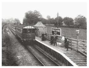
use of corrugated iron as a building material. An example at GWR of this was the elegant and efficient 'pagoda-style' shelter utilised at Stanley halt as in this picture taken in 1905. Pagoda shelters were relatively simple prefabricated structures, to a standard design. They were later simplified further to a simple box shelter.
