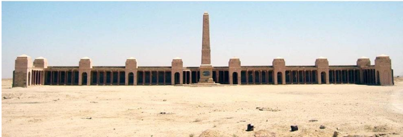
The Basra Memorial, The original and The Rebuild
